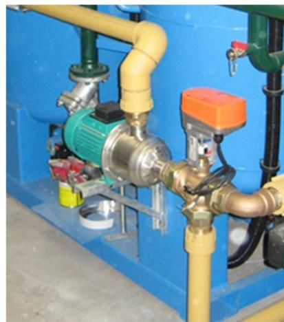
Figure 16: Problems with three-way-valve, office building in Rohrbach, Austria
